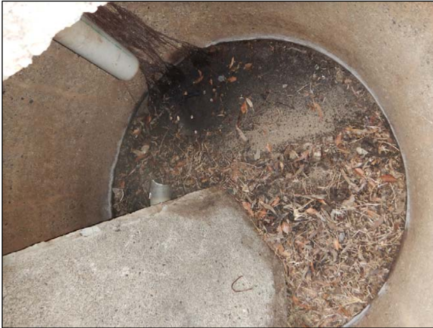
Figure 13: View of inside of concrete septic tank
