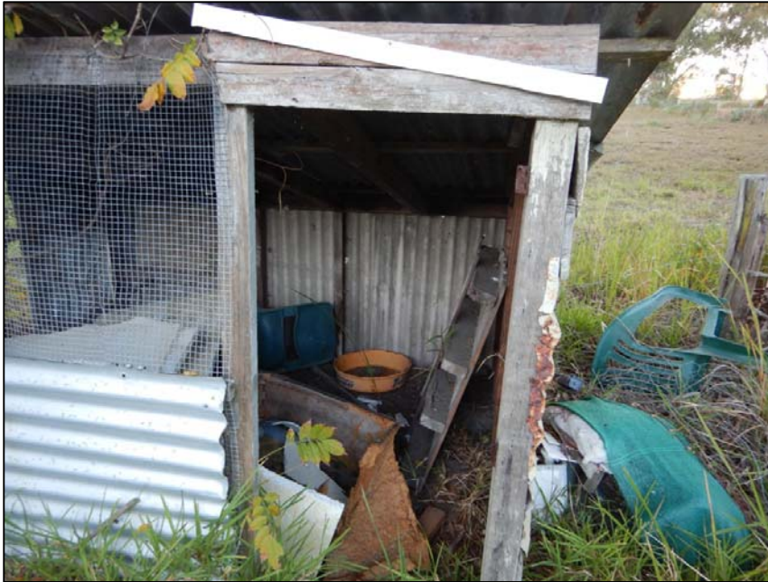
Figure 9: View of small shed with fibro sheeting (possible ACM) on walls
